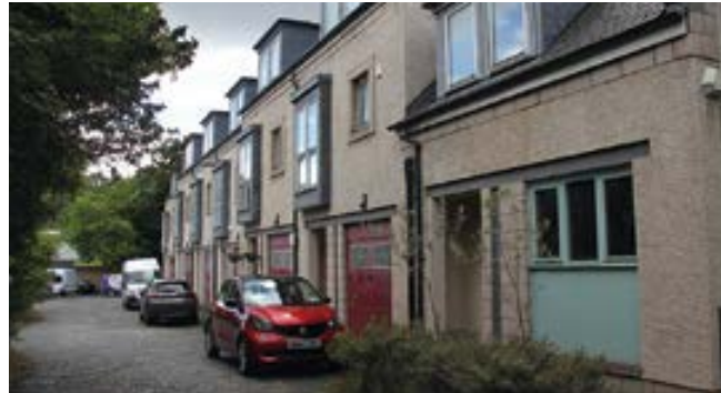
Mix of integral garages and on-street parking within the mews development at Eyre Place
