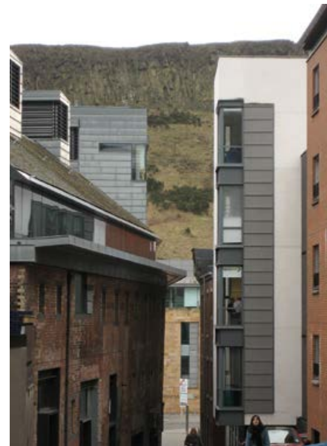
Creating new views - Jackson's Entry off Canongate Views to Salisbury Crag are framed by the retained historic buildings and the new development that resulted from the masterplan.
