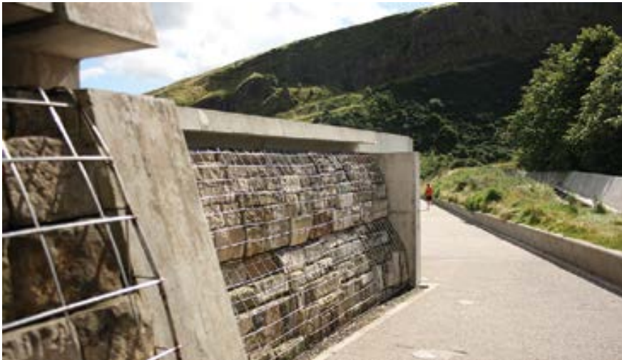
Reusing building materials—Holyrood Road Stone from the partially demolished Queensberry House was used in the walls on the exterior of the Scottish Parliament.
