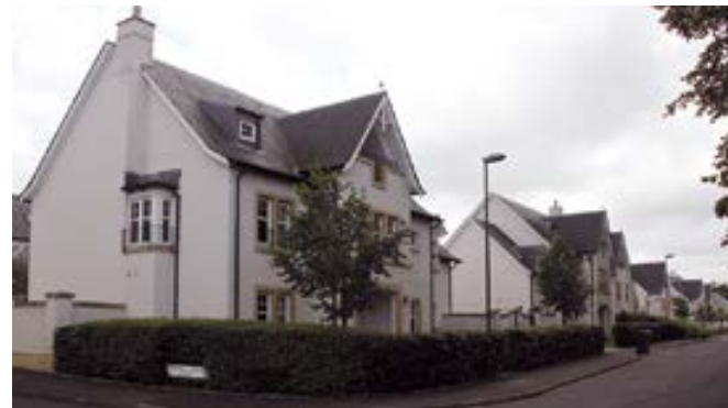
Dwellings at Redhall House Drive pushed forward on the plot with strong boundary treatment and defensible space to the front
