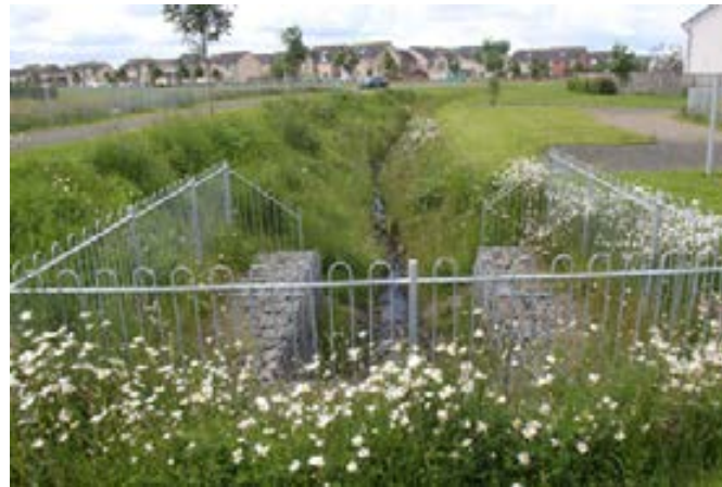
SuDS retention basin and swales, Kirkliston
